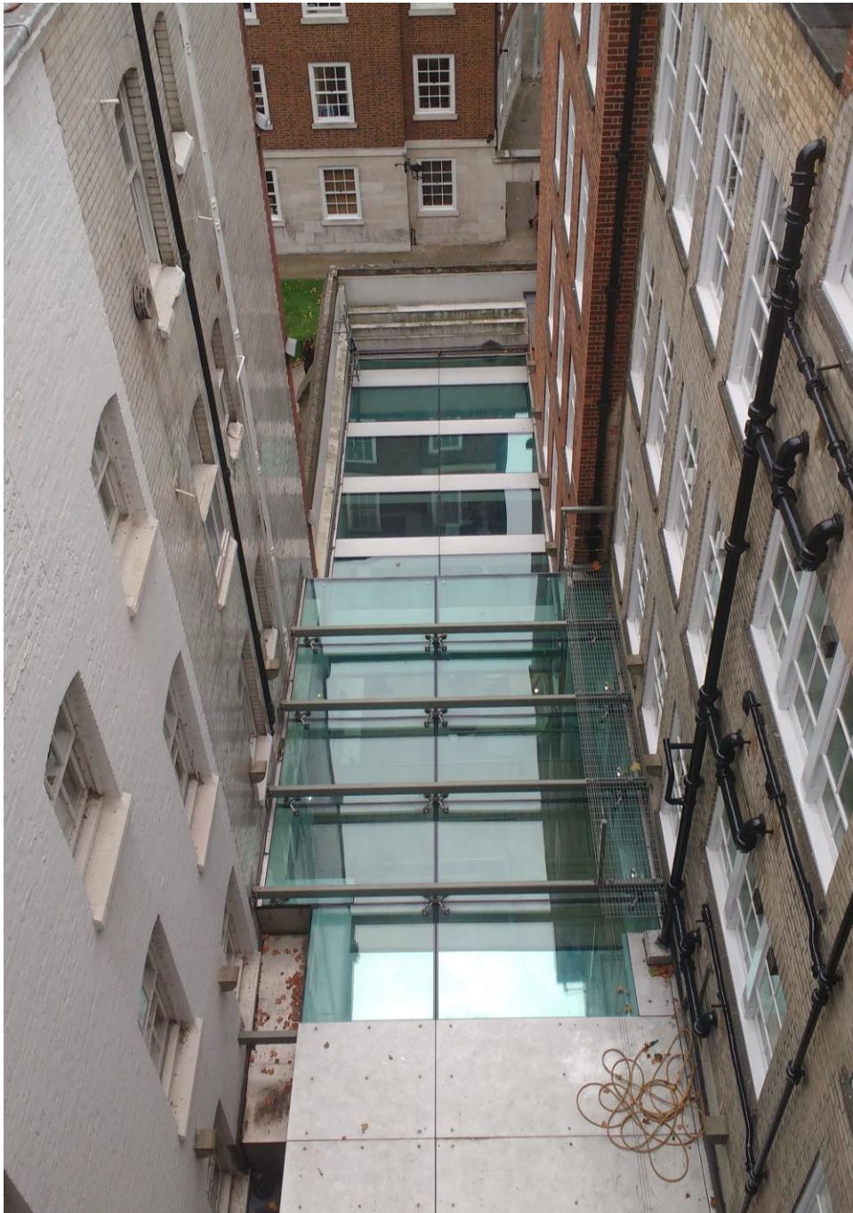
View from fire escape Blackstone House (right) and 1 & 2 Garden Court (left)
